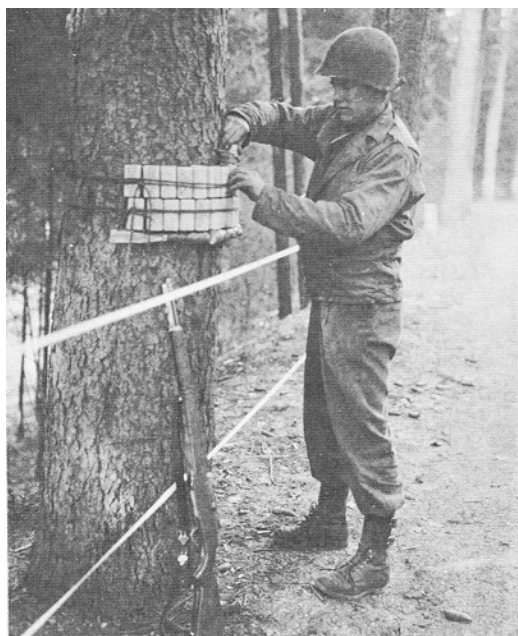
COMBAT ENGINEER SETTING A CHARGE.
